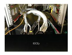
In the next step install the IEICEy in the centre mounting rail of the rack. Again this 19" chassis can be wired from the front and then inserted as shown on the picture in the left.
